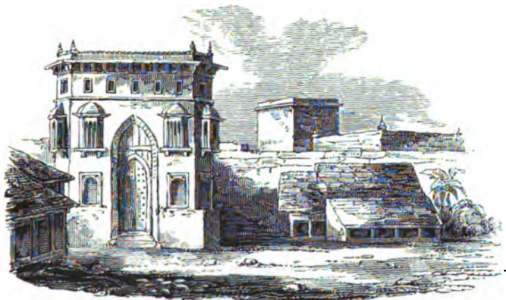
GOTHIC GATEWAY AT GHAZIPOOR
